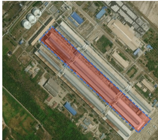
Figure 1. Aerial view of INALUM’s reduction plant.
