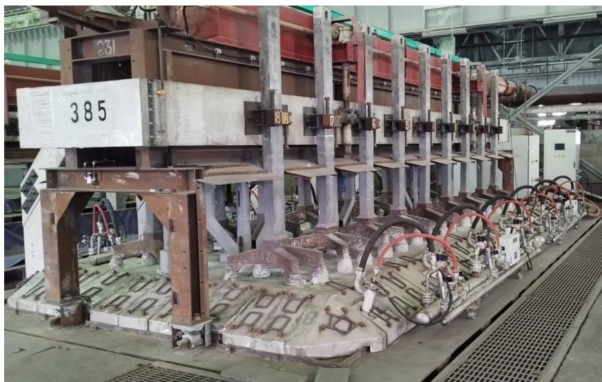
Figure 5. Preheating process preparation.
